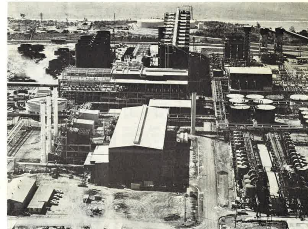
The alumina plant, almost ready to commissioning.
